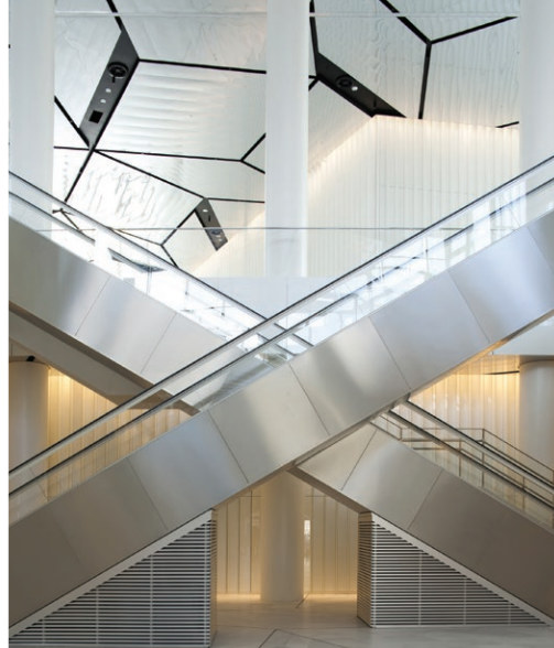
Ceiling, Allianz Tower, Milan (I) Colombo Costruzioni S.p.A., arch. Isozaki
